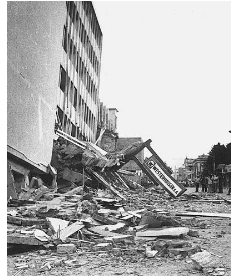
Collapse of a hotel during an earthquake in El Salvador in 1986
